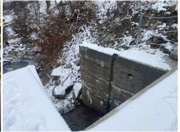
November 2021 – Right wall of Outlet Flume
