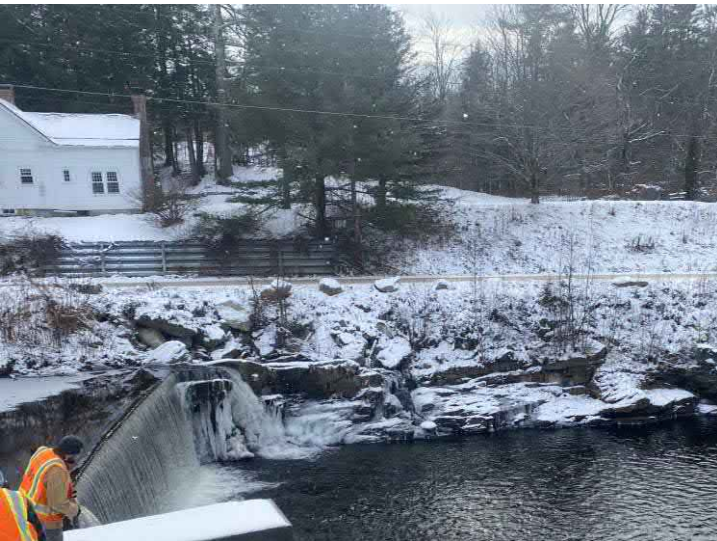
November 2021 – Left Abutment
