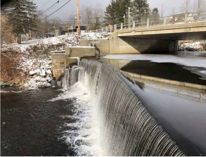
November 2021 – Primary Spillway
